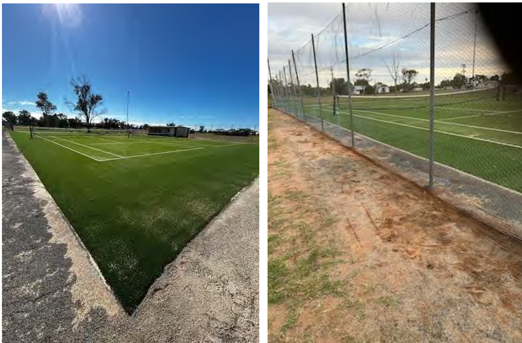
Figures 1 and 2: Completed Quambone Courts with fence reinstated
